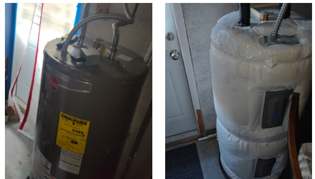
Water Heater Wrap: Before and After
